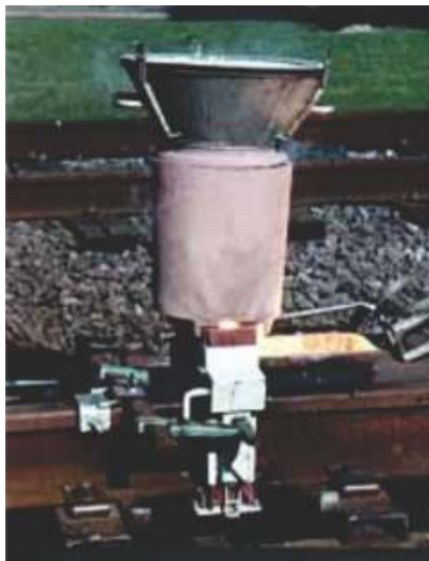
Fig. 7.09 Single shot crucible
