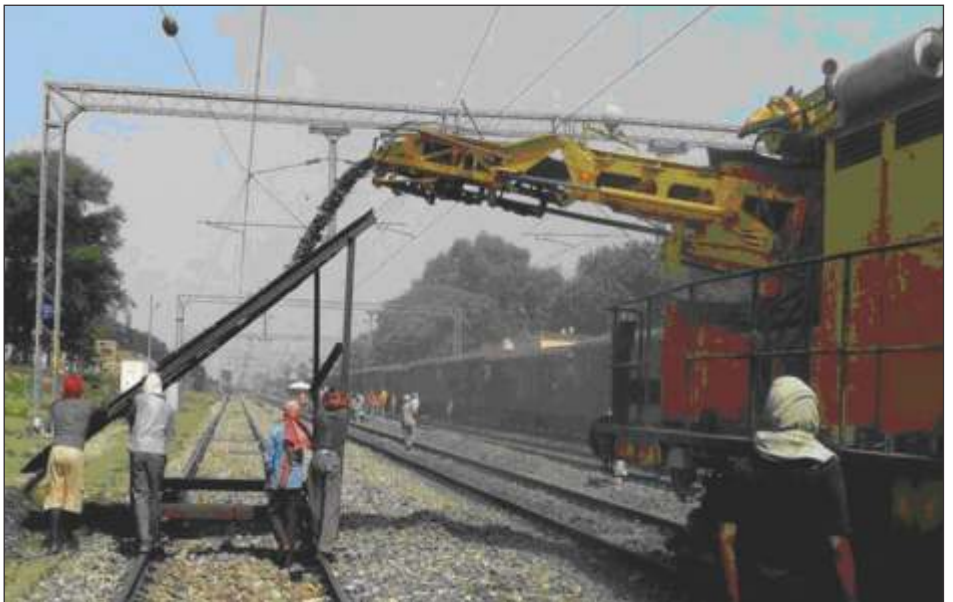
Fig. 10.02 - Arrangement for soil disposal from Ballast Cleaning Machine.
