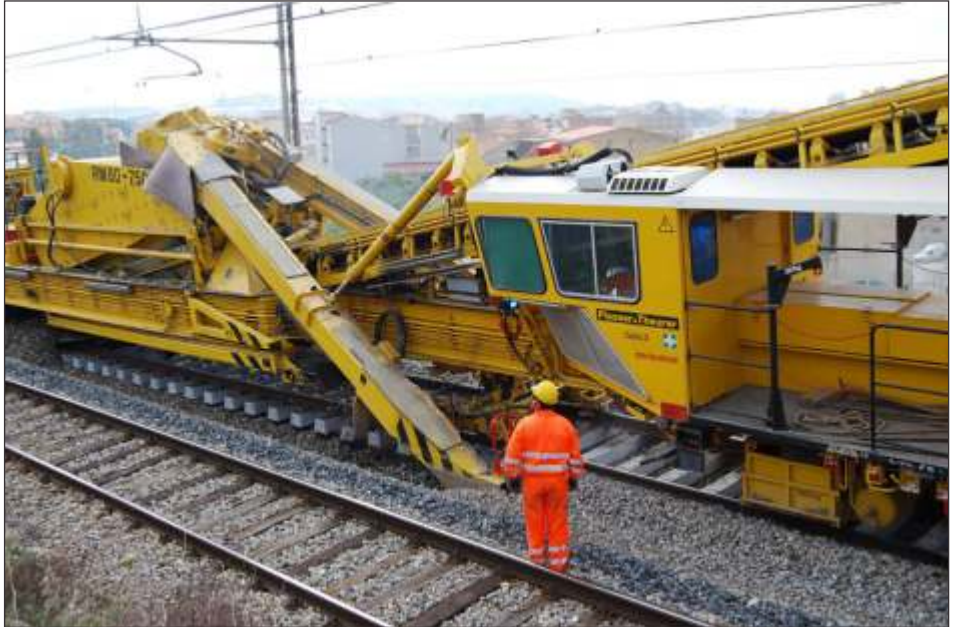
Fig. 10.03 Deep Screening of Ballast by BCM
