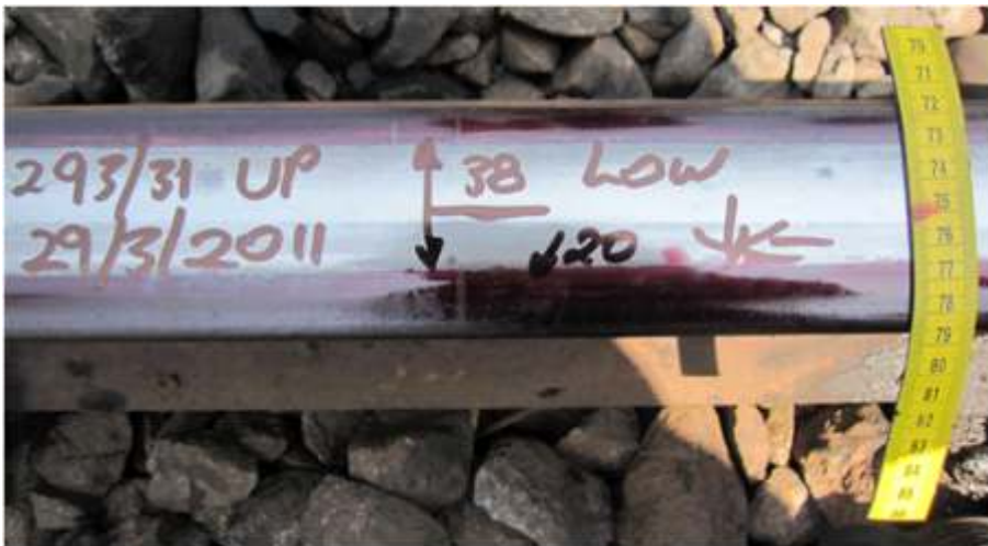
Fig. 8.40 - Photograph showing contact band details after grinding
