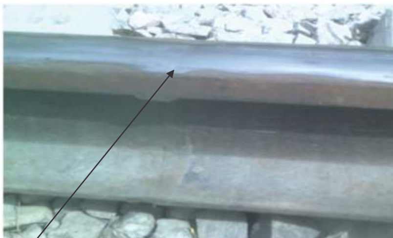
Flash Butt Welded Joint
